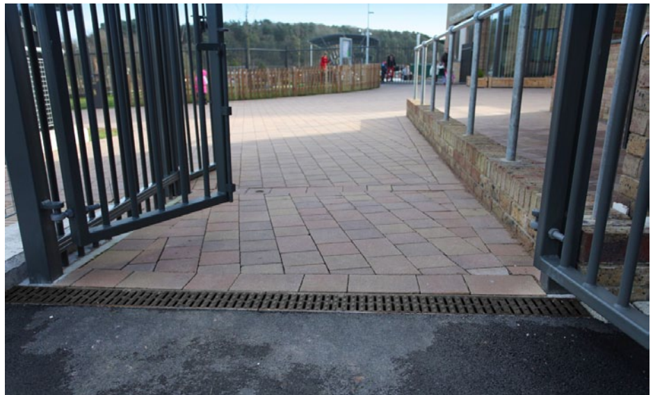
ACO MultiDrain M100D was used at various points across the site to provide surface water drainage.
