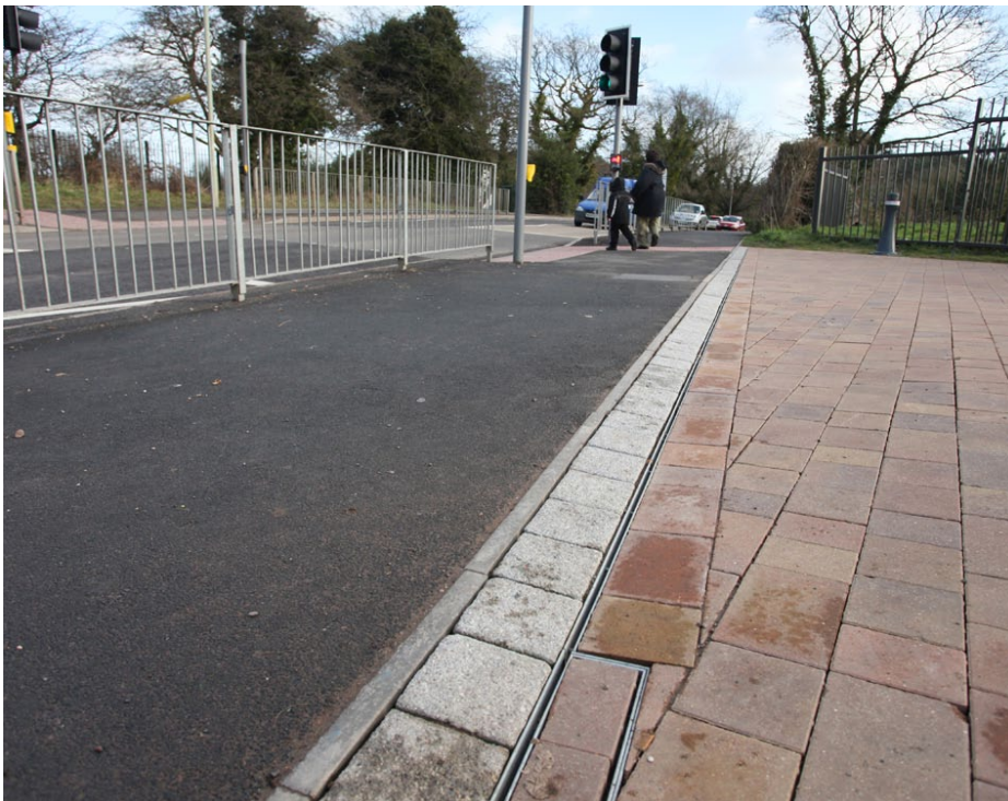
ACO MultiDrain Brickslot provides discreet slot drainage to hard landscaped areas.
